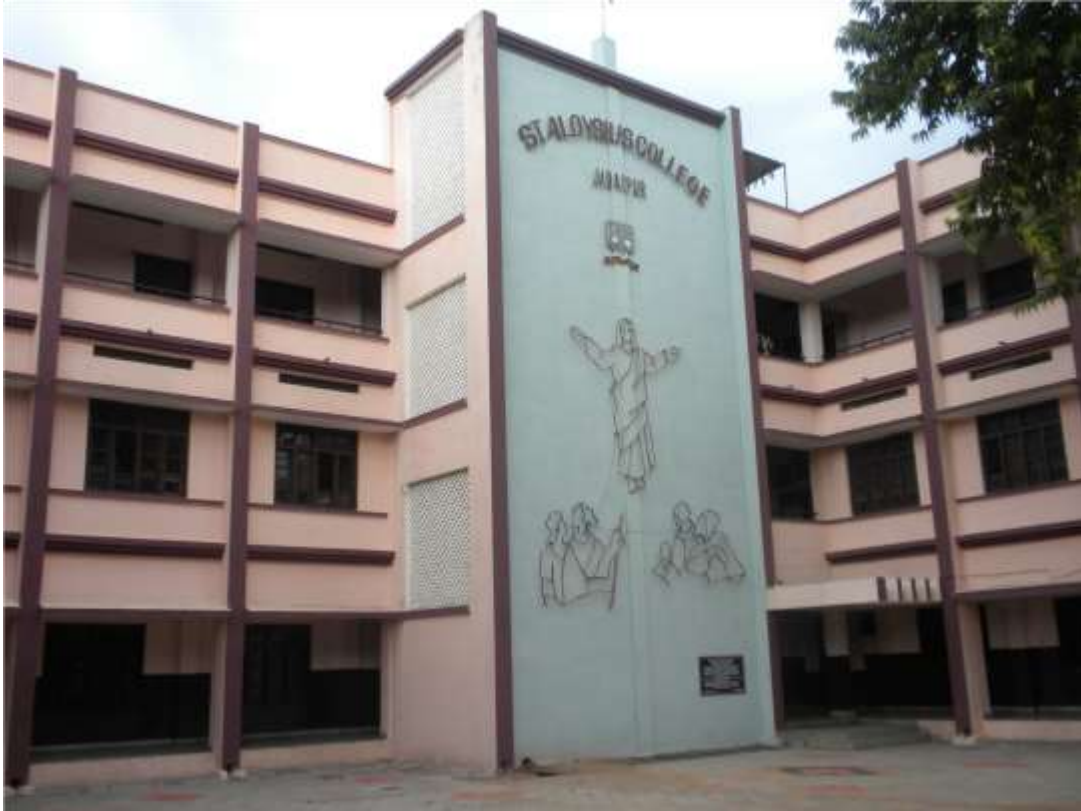
Rear view of the building
