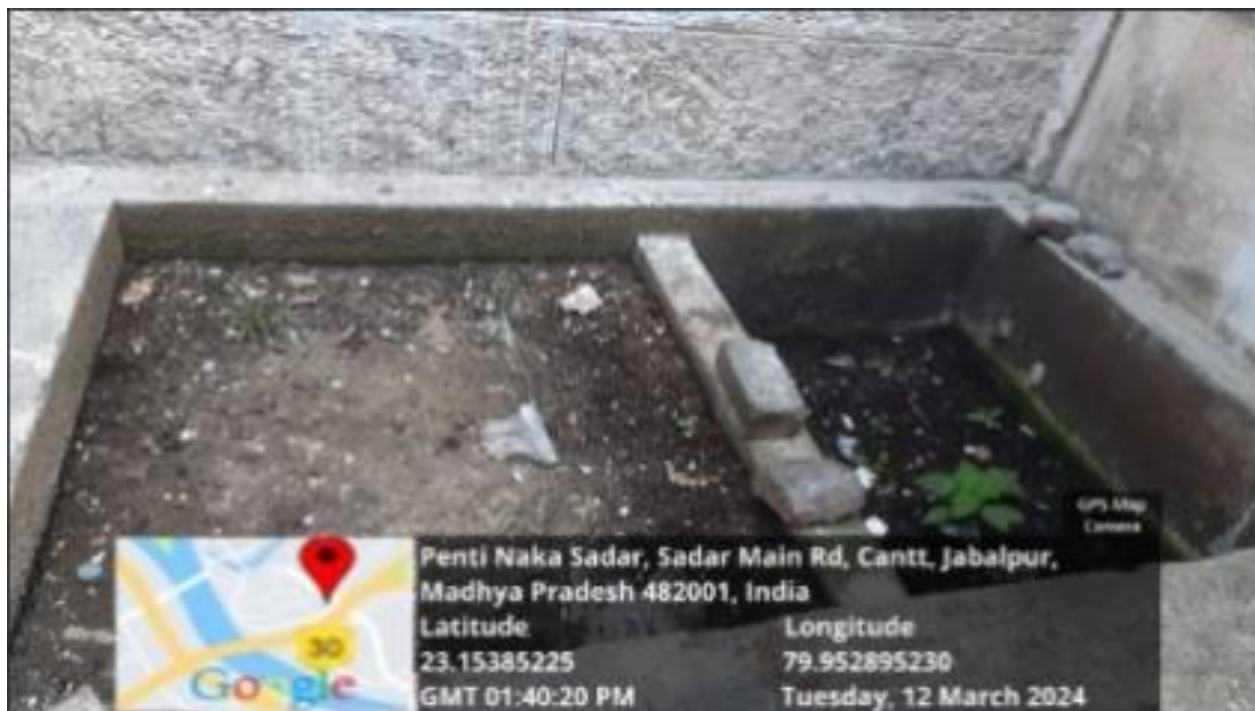
Plate 1: Compost pit in the premises
