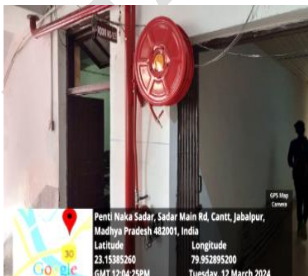
Plate 5: Fire hose reel and extinguisher in the premises
