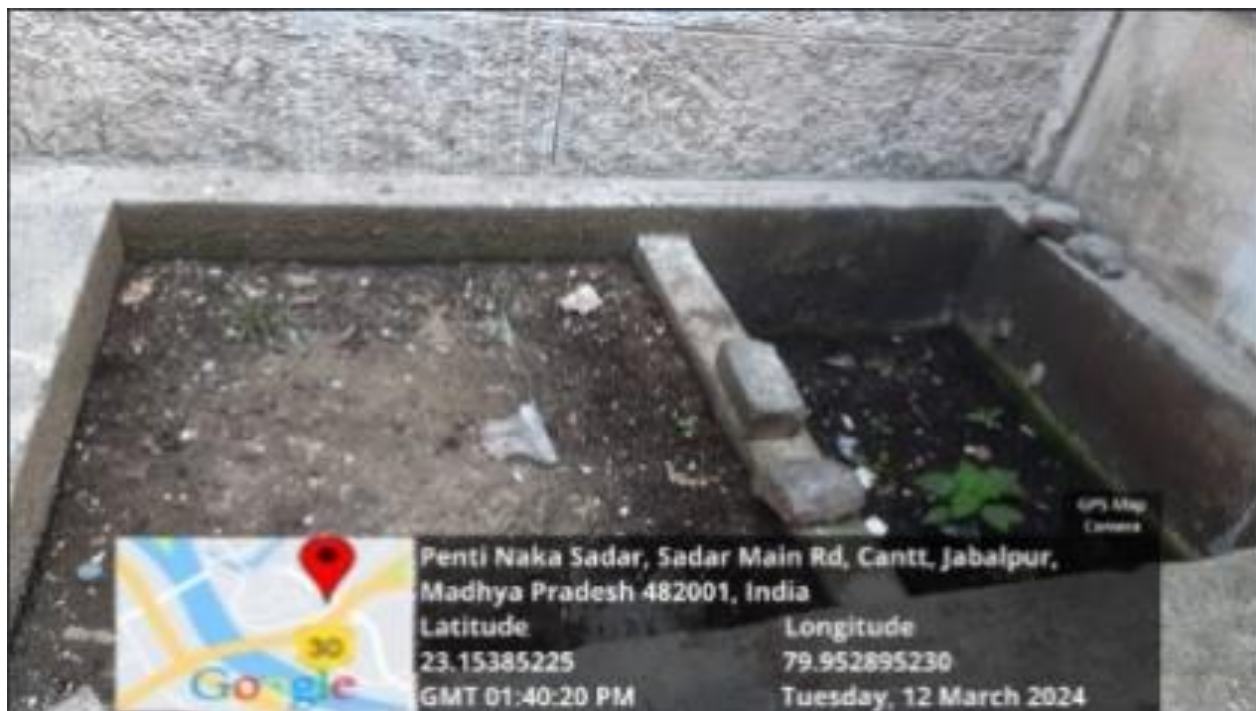
Plate 1: Compost pit in the premises
